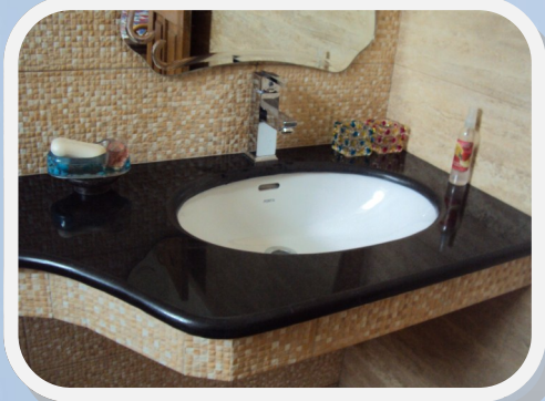
Renovation work F-11/3
