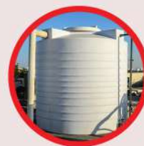
Water Tank Cleaning
